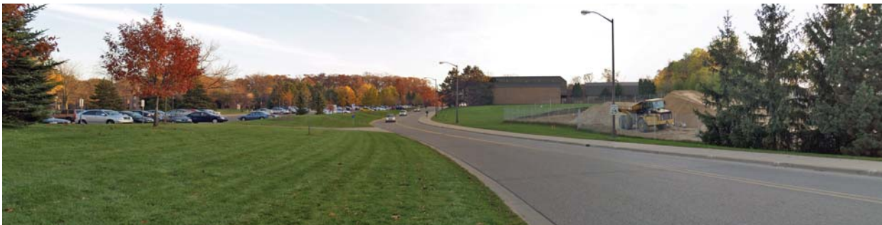
Existing conditions at the Murfin Avenue- Plymouth Road intersection, looking south
