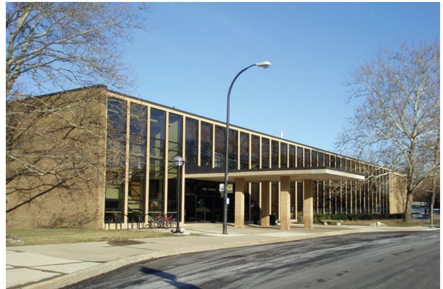
Cooley Building (built in 1953)
