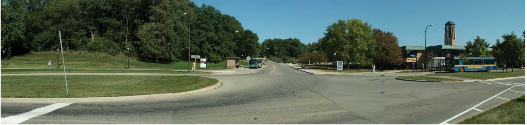
Existing Bonisteel - Murfin intersection, view north
