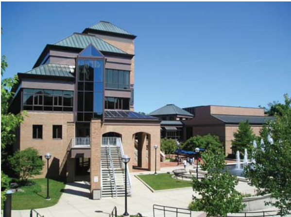
Lurie Engineering Center
